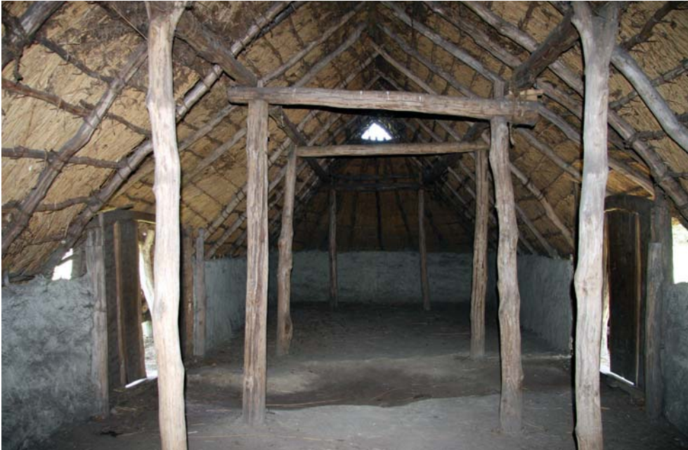
Figure 6.4 Reconstruction of an Iron Age farm at Orvelte (Netherlands) which shows the structure of the farm, including the roof cover, the battens and the rafters resting on purlins and on the wall plate (on top of the walls) (photo: H. Fokkens).
