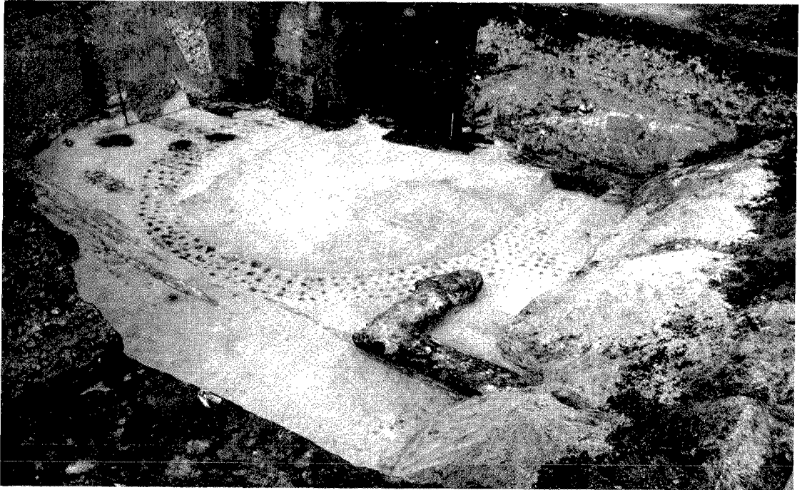
1 Aardenburg: detail of pile foundations under a Roman building from the late second or early third century ( cf. fig. 4a); excavation ROB 1961-3
