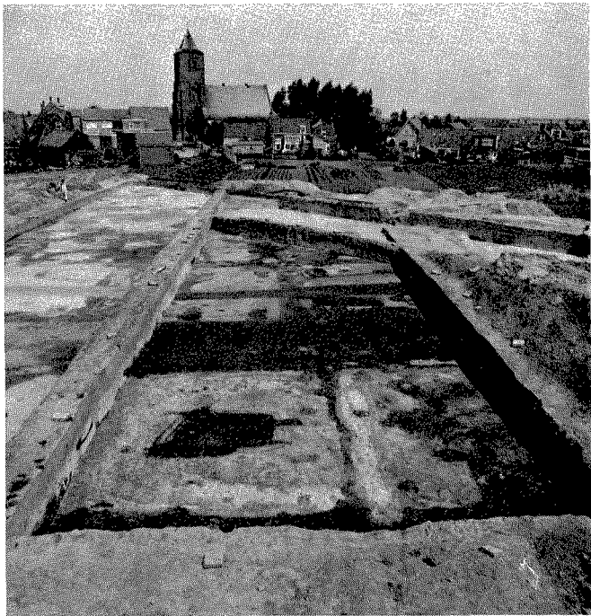
1 Survey of the excavations of 1969. In the background the parish church of Oost-Souburg
