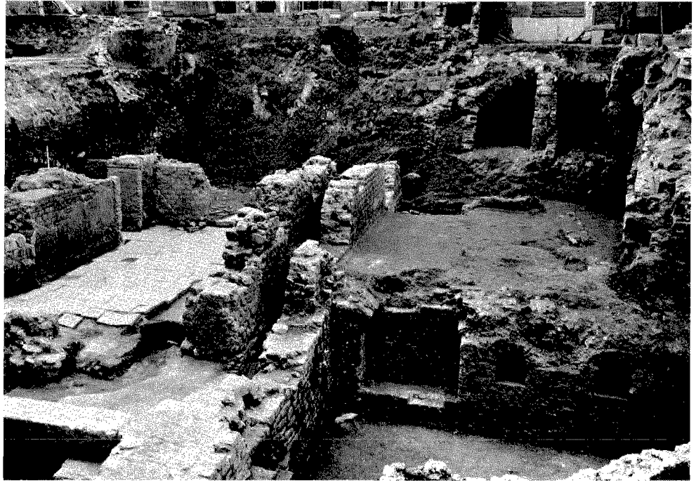
1 Maastricht, Stokstraat area: Thermal baths from the east, September 1963
